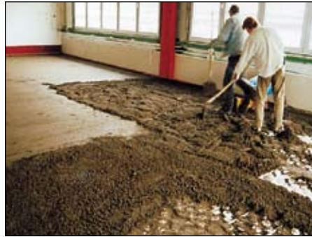
A dry-pack mortar screed (on the left) or poured gypsum screed (on the right) is placed over the Schluter®-BEKOTEC modular screed panel and hydronic radiant heating tubes without control joints or wire reinforcement.
