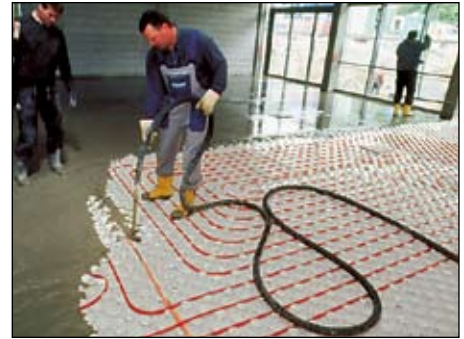
A dry-pack mortar screed (on the left) or poured gypsum screed (on the right) is placed over the Schluter®-BEKOTEC modular screed panel and hydronic radiant heating tubes without control joints or wire reinforcement.
