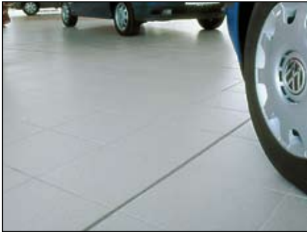
Ceramic tile installed over the Schluter®-DITRA uncoupling membrane and Schluter®-BEKOTEC modular screed system in an auto showroom.
