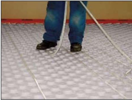
Hydronic radiant heating tubes are conveniently placed between the studs of the Schluter®-BEKOTEC modular screed panel without clamps before the screed application.
